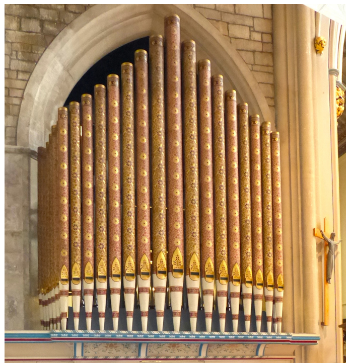
Image 5 | Nave case pipes before restoration
